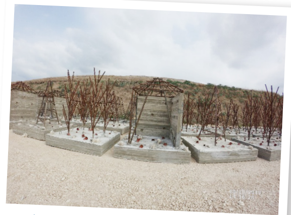
Figure 2. AR2020 units under construction (Source: MCR-IOE-UOB)
